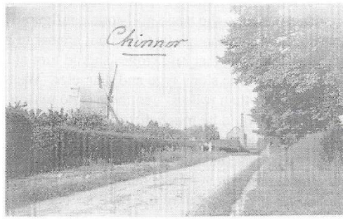
Chinnor steam and wind mills some time after 1900 Note patent sails and fantail on windmill, and brick chimney on steam mill house
