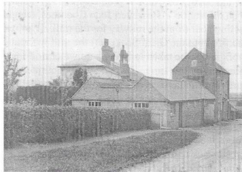
Chinnor steam mill some time after 1900. The boiler/engine was housed on the nearest side of the chimney. Coal was stored in this low building too. In the foreground was the office with a store room behind it. The feed hoppers were in the roof of the main steam mill building nearest the chimney. The Mill House is the white building to the rear of the steam mill.
