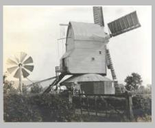
By 1903 it had been upgraded with all the latest technology: a fan tail that automatically keep it pointing into the wind, and automatic 'Patent' sails which adjusted themselves to suit different wind strengths
