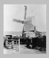
Originally the Miller would have turned the whole mill on its post, to keep it pointing into wind, and continuously adjusted the cloth sails, folding them back in strong winds
