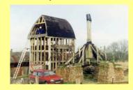
The 'buck' was built alongside the post to reduce the amount of working high up on scaffolding, and in 2011 the buck was finally lifted onto its post by a 70 ton crane.
